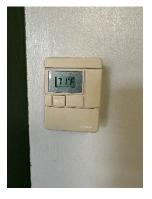
3. Plans should be made to upgrade the older Siemens control system with the newer Siemens/Desigo system to be consistent with the rest of the district. At that time, the standalone electric thermostats and controls serving the cabinet heaters and convectors would be replaced with new digital sensors and control components tied back to the central BAS.
